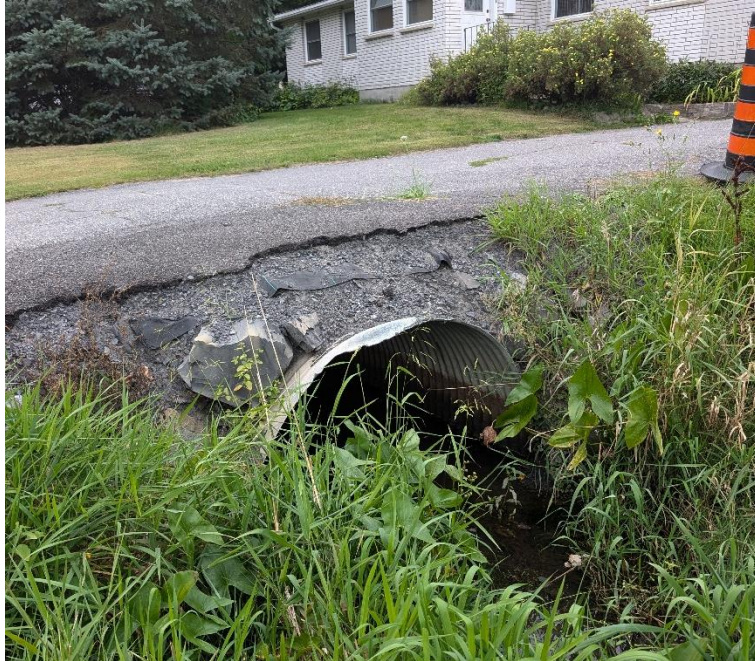
Figure 15: Downstream end of the enclosure at station ±8+66 that crosses Clarence Street
