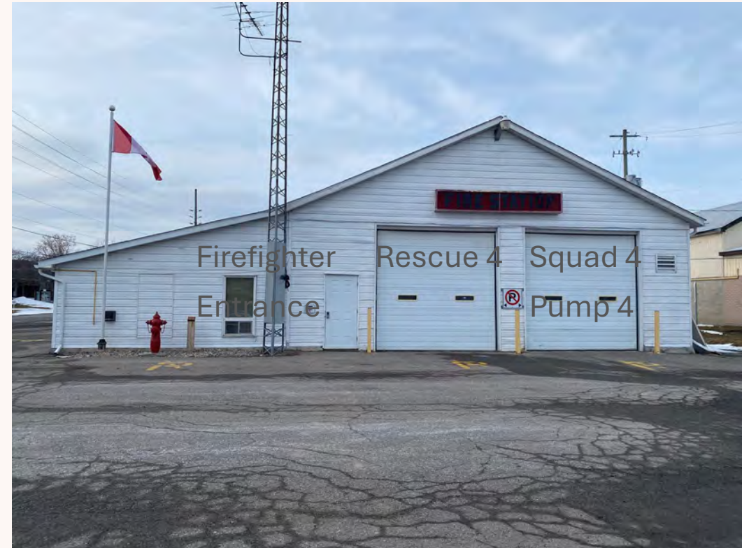
South side of building
