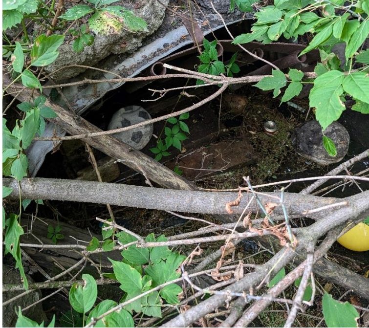
Figure 21: Showing CSP culvert crossing Queen Street on Main Drain at station \pm 13+63 . Significant debris and vegetation were noted at both ends. Measured 48" across.
