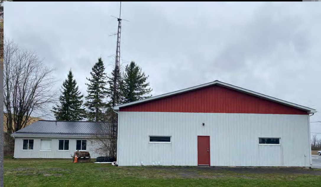
West side of building - Rear
