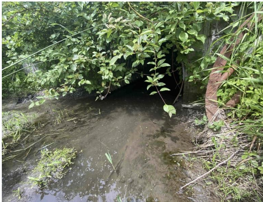
Figure 14: Upstream end of the enclosure at ±7+99 that crosses Clarence Street.
