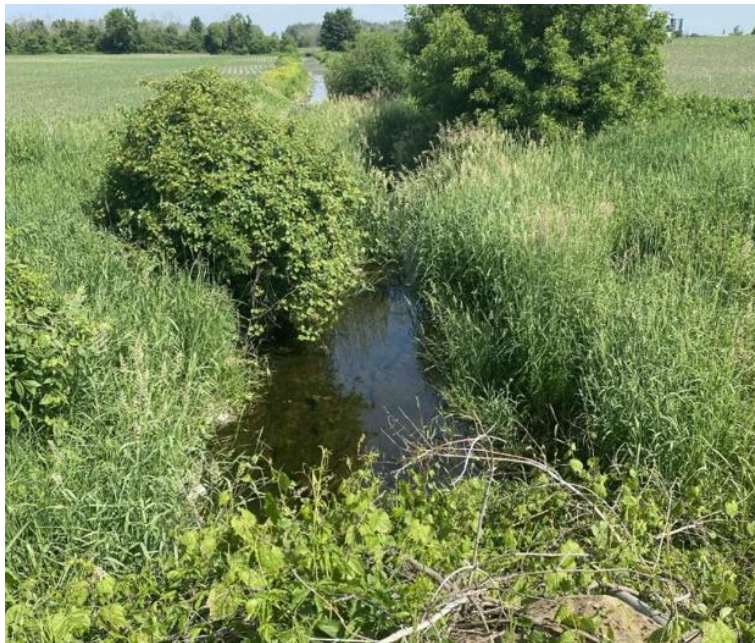
Figure 28: Looking downstream from culvert at Station ± 37+20.
