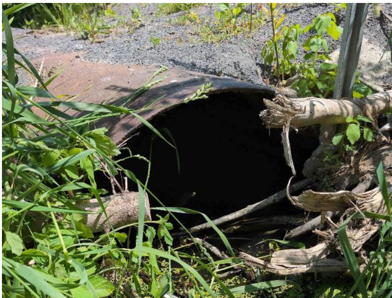
Figure 26: Showing an example of a farm crossing culvert on the Diversion Drain made from non-standard materials, located east of Queen Street and Lancaster Lane.
