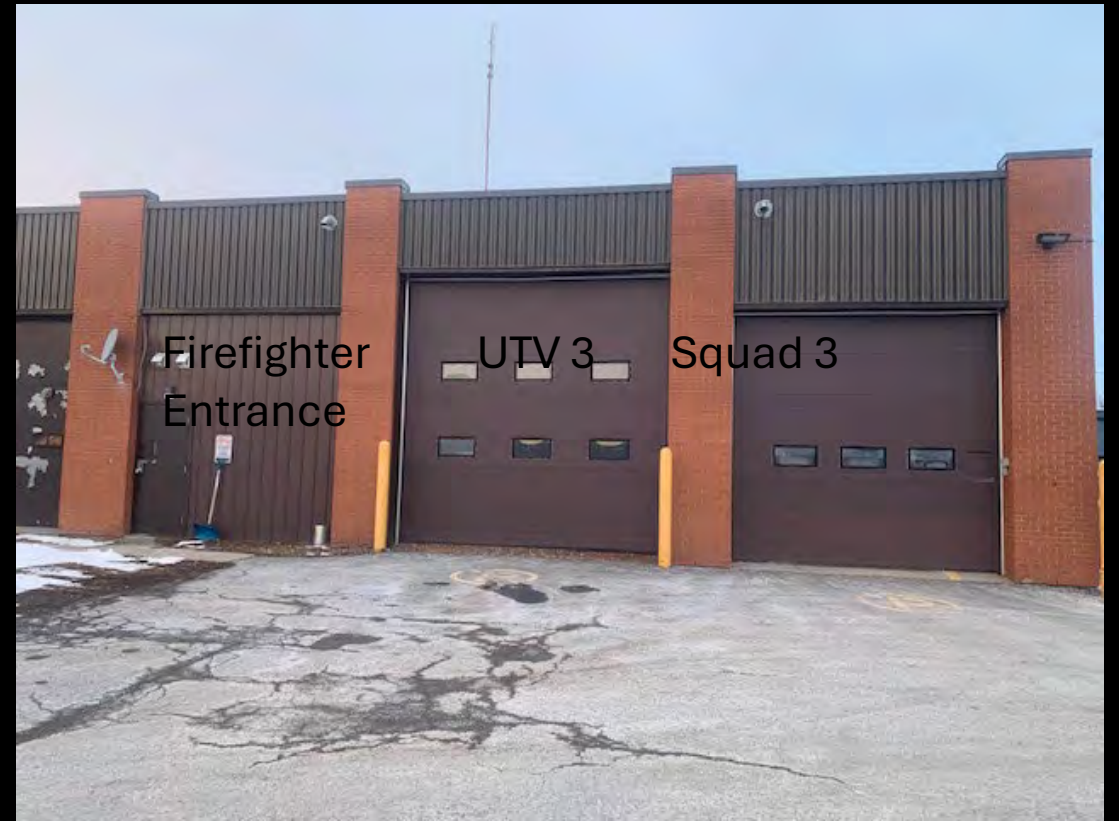
South side of building
