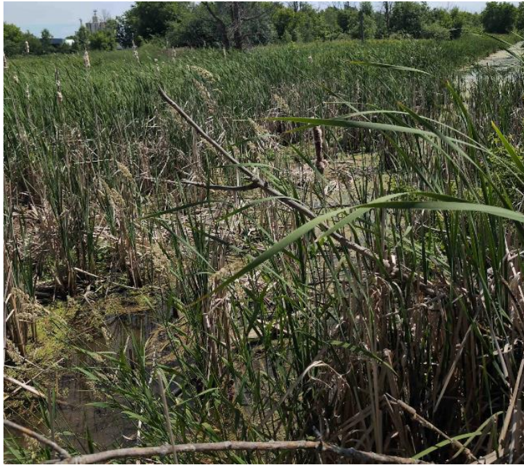
Figure 1: Significant vegetation growth observed between stations 0+00 and ±1+89. The example shown near upstream limit of Henderson Creek Municipal D rain.
