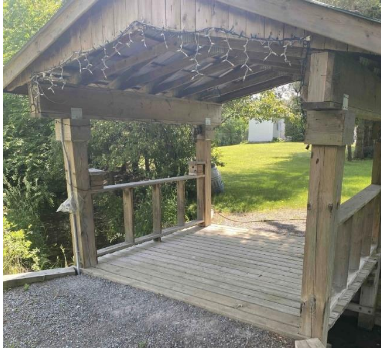
Figure 3: Example of a footbridge over the drain in the section between stations \pm 3+06 and \pm 3+97 .
