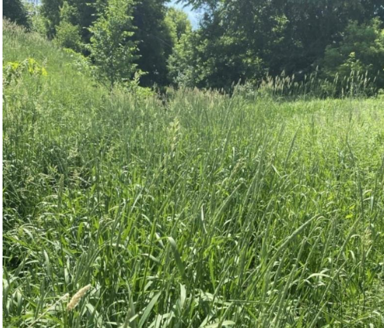
Figure 25: Showing heavy vegetation growth in the section of drain adjacent to the wastewater ponds at station ±22+80.
