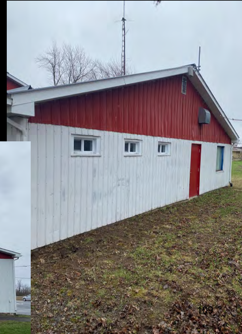
South side of building
